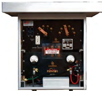
RM4150 Placed in Rectifier
