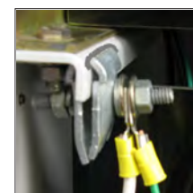
RM4015 Ground Connection to I-beam Ground Clamp
