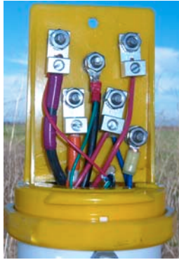
Figure 2-17. Test Station Terminal Board - After Installation
