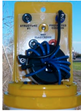
Figure 2-17. Test Station Terminal Board - After Installation
